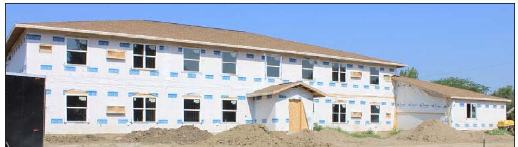
HRC apartment building - on the old hospital building site.
